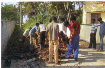
Drainage cleaning work
